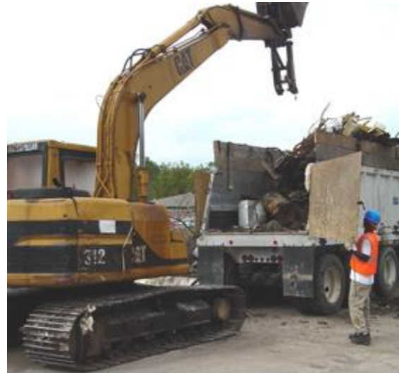
Photo courtesy of OSHA. This picture shows actual disaster site work
